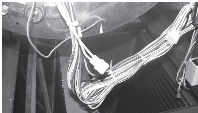
Figure 11: Remove Harness Plug
