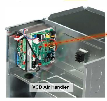
S1/S2 Output to Outdoor Unit (Polarity Sensitive)
